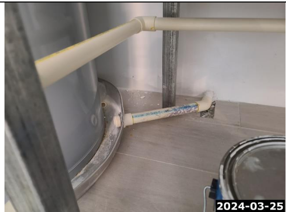
Water Heater Drain
