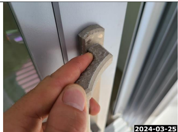
Visible Corrosion Noted at Exterior Door Handles
