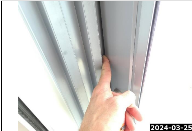
Movement at Door When Latched – Door Opens About ¼ inch When Locked
