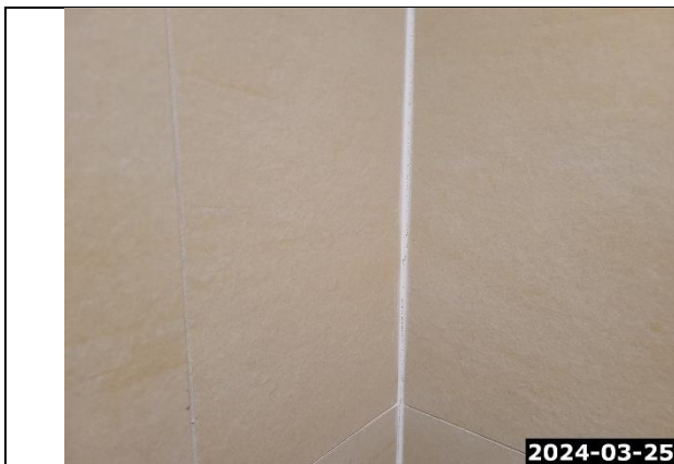
Bathroom #1 Cracking at Caulk
