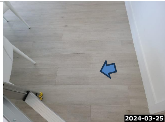
Tile Grout Damage at Main Walk / Hallway
