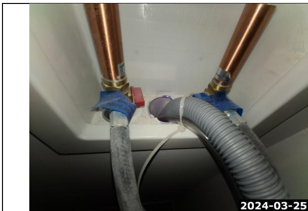
Laundry Plumbing Supply Valves
