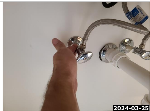
Bathroom #2 Movement at Supply Line
