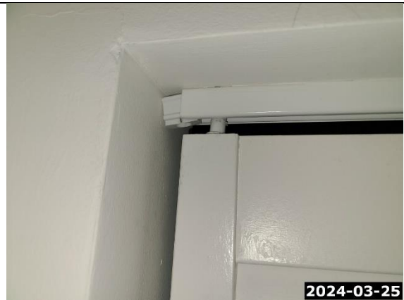
AC Closet Door Track Service (Inside Utility Room)
