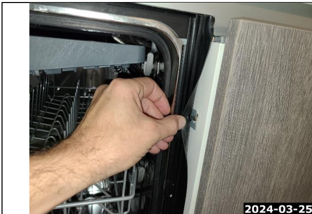
Dishwasher Attachment Screw Crooked
