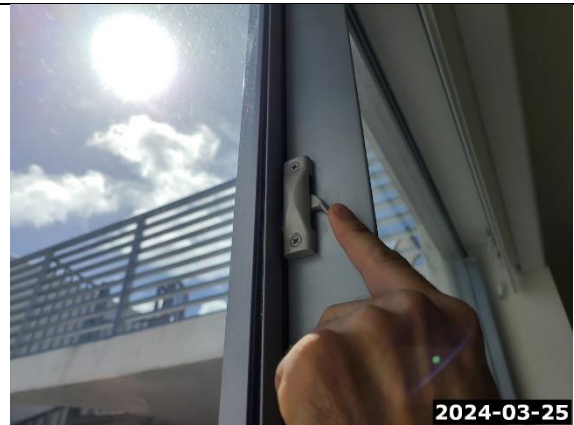
Lock Not Latching at Window
