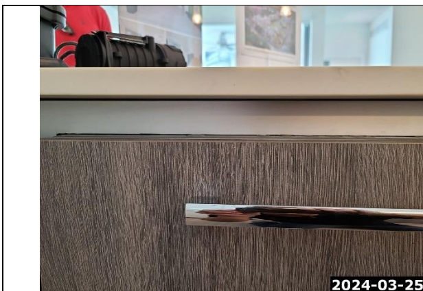
Dishwasher – Buttons in Contact with Cabinet
