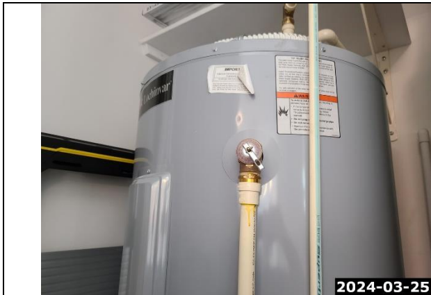
Water Heater Relief Valve (TPRV)
