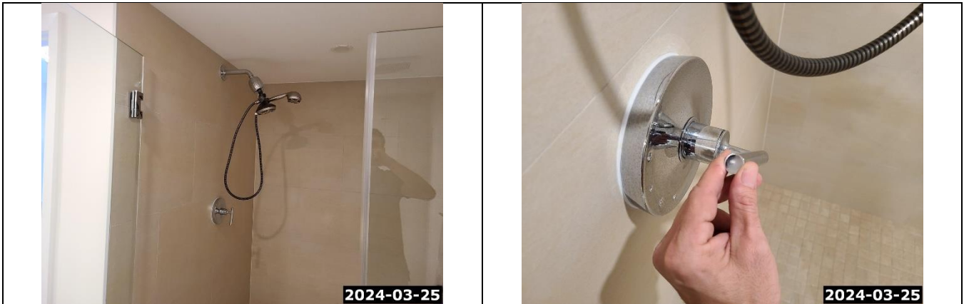
Bathroom #3 Images Bathroom #3 Movement at Shower Handle
