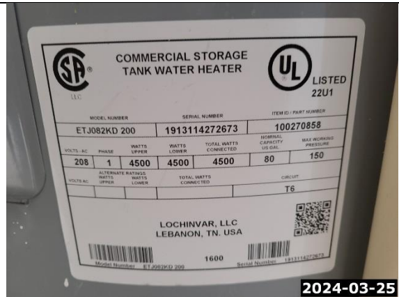
Water Heater Manufacturer's Label
