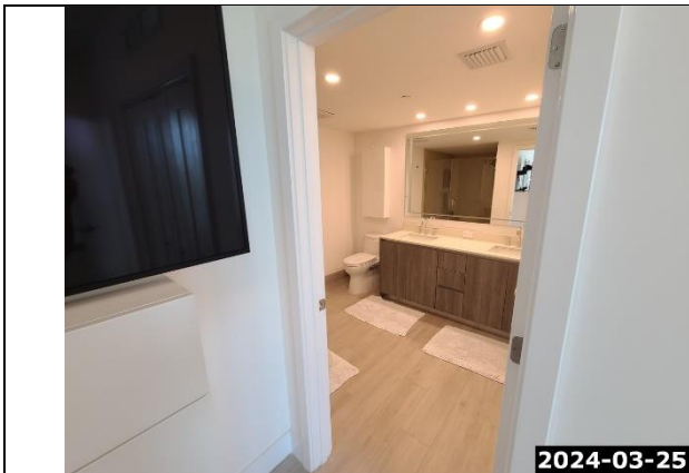
Loose Door Handle (Master Bathroom as Example)
