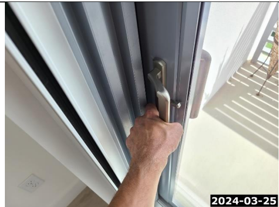
Movement at Door When Latched
