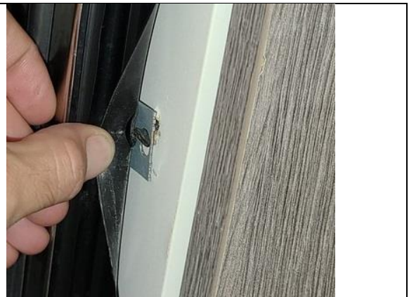
Dishwasher Attachment Screw Crooked
