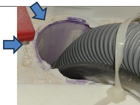
Damage at PVC at Laundry Supply Box
